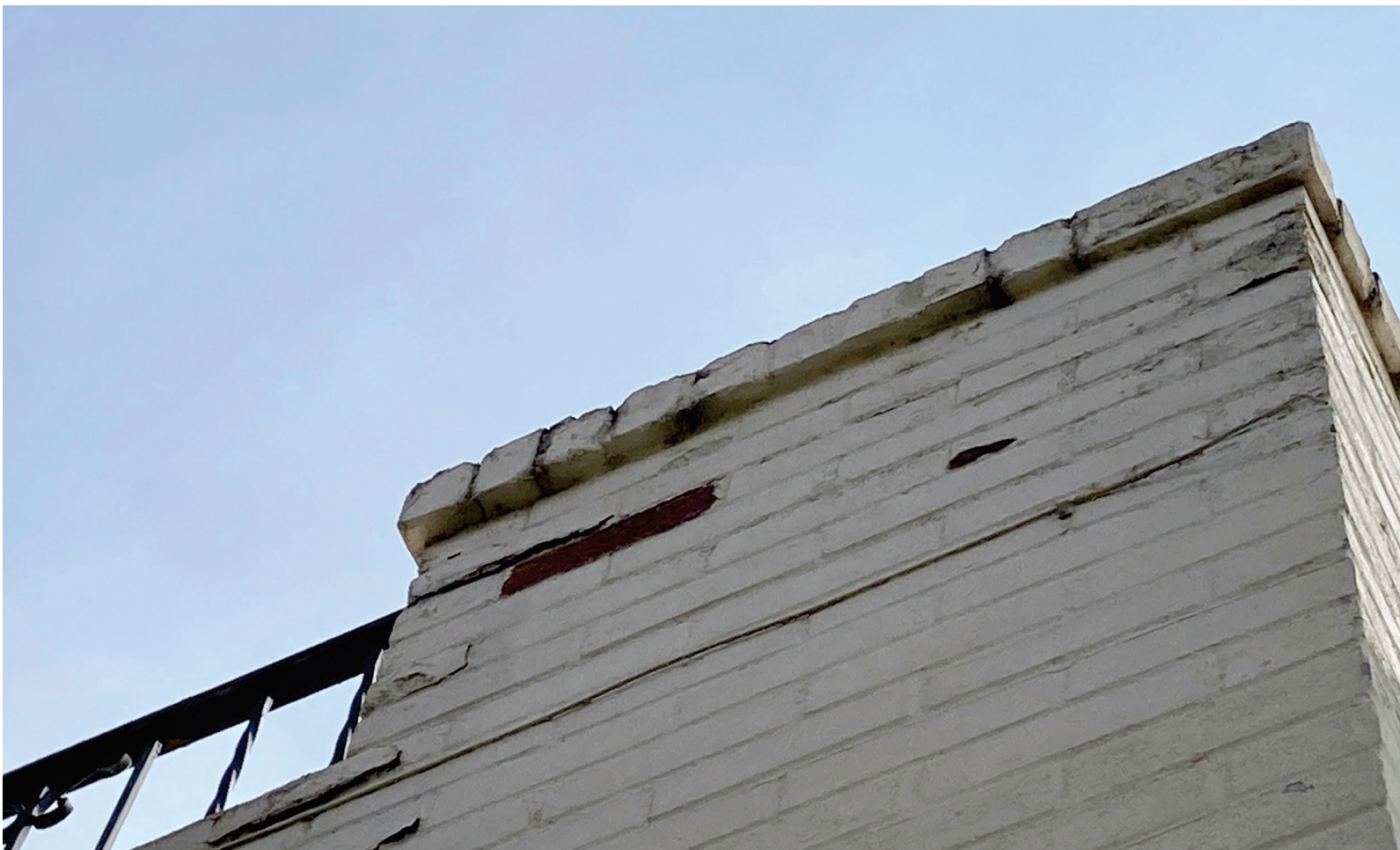
SPALLED WEST PARAPET
