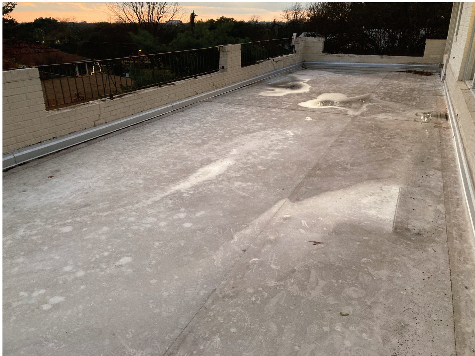
PONDING THROUGHOUT ROOF AREA
