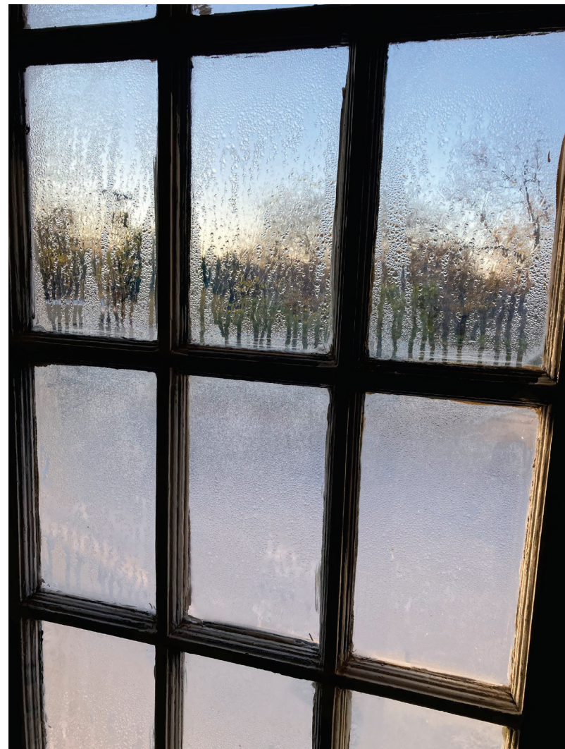
TYPICAL INTERIOR INFILTRATION & CONDENSATION
