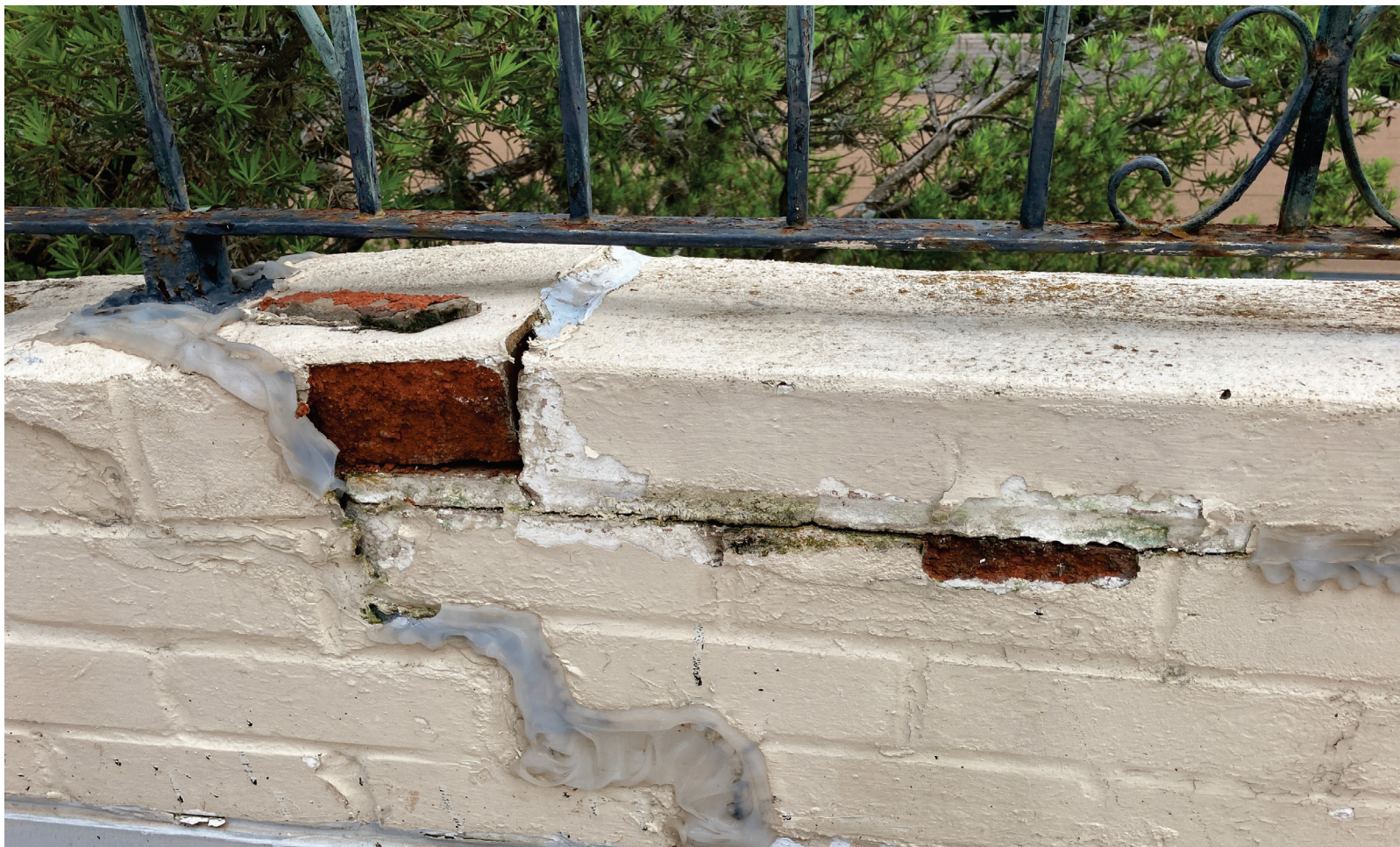
DISPLACED BRICK OVER CANOPY
