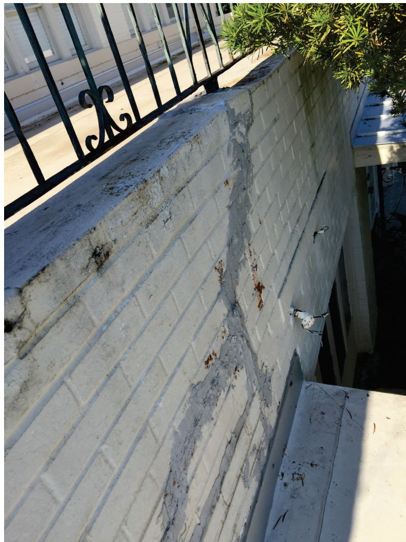
BRICK DISPLACEMENT @ CANOPY
