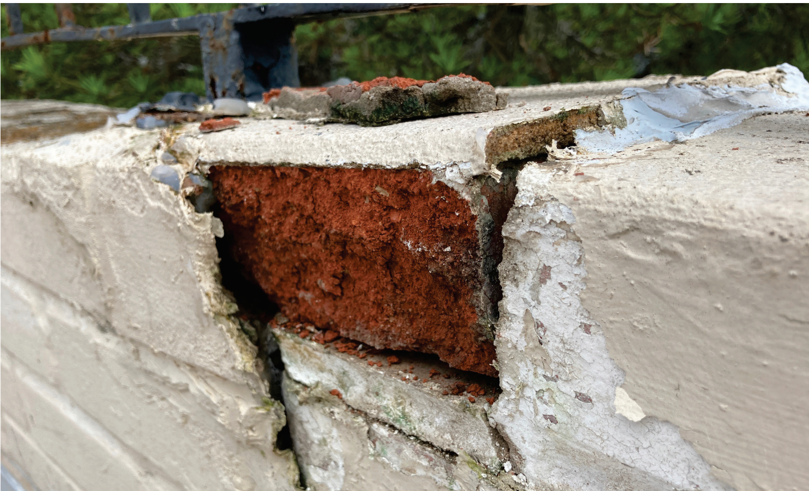
BRICK DETERIORATION & CRACKING
