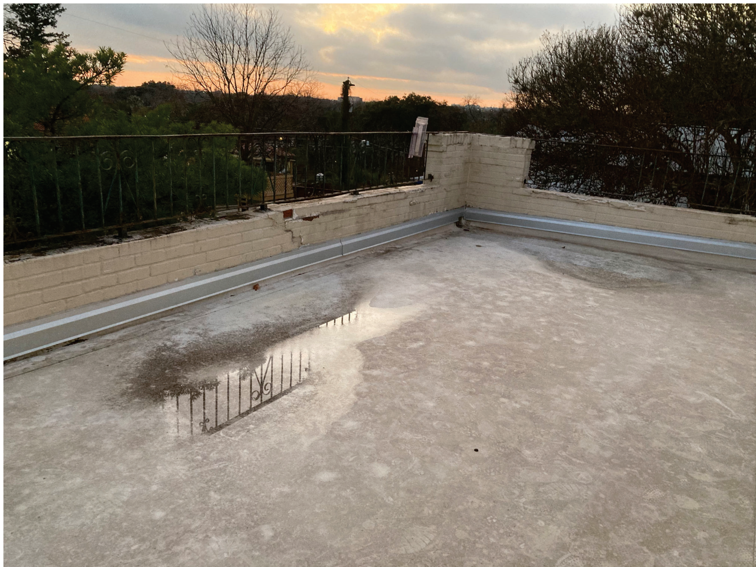
TYPICAL PONDING DUE TO INSUFFICIENT SLOPE
