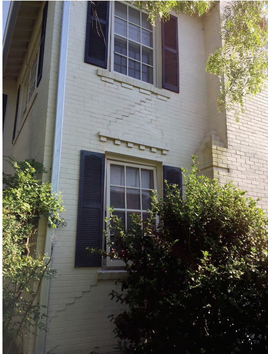
TYPICAL MASONRY CRACKING @ NORTHEAST
