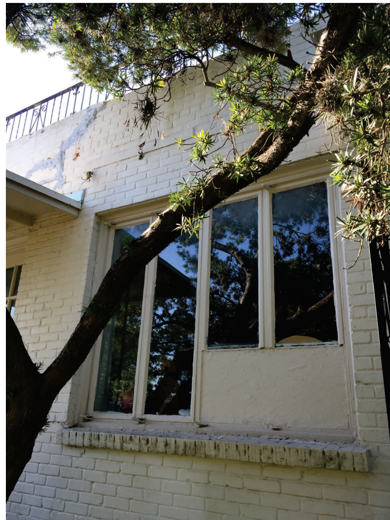
FAILED STEEL CASEMENT
