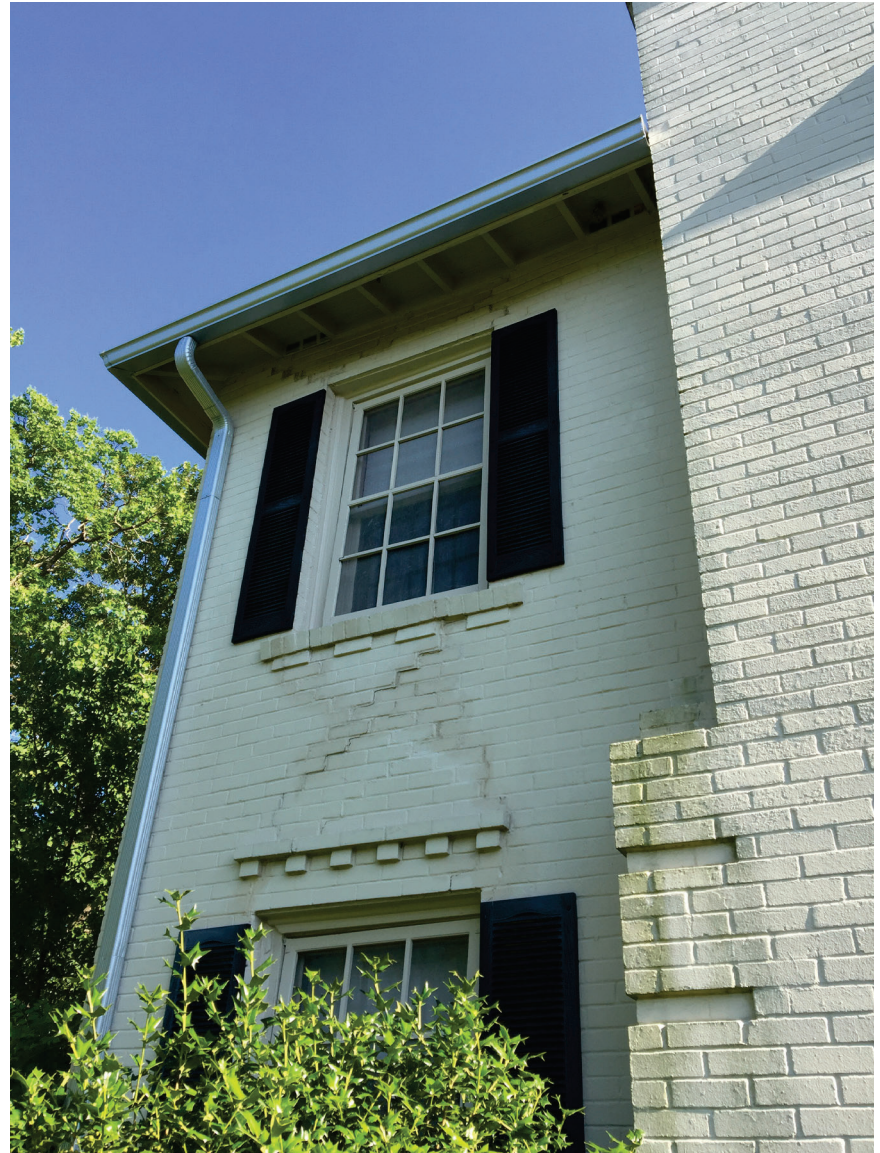
TYPICAL MASONRY CRACKING @ NORTHEAST
