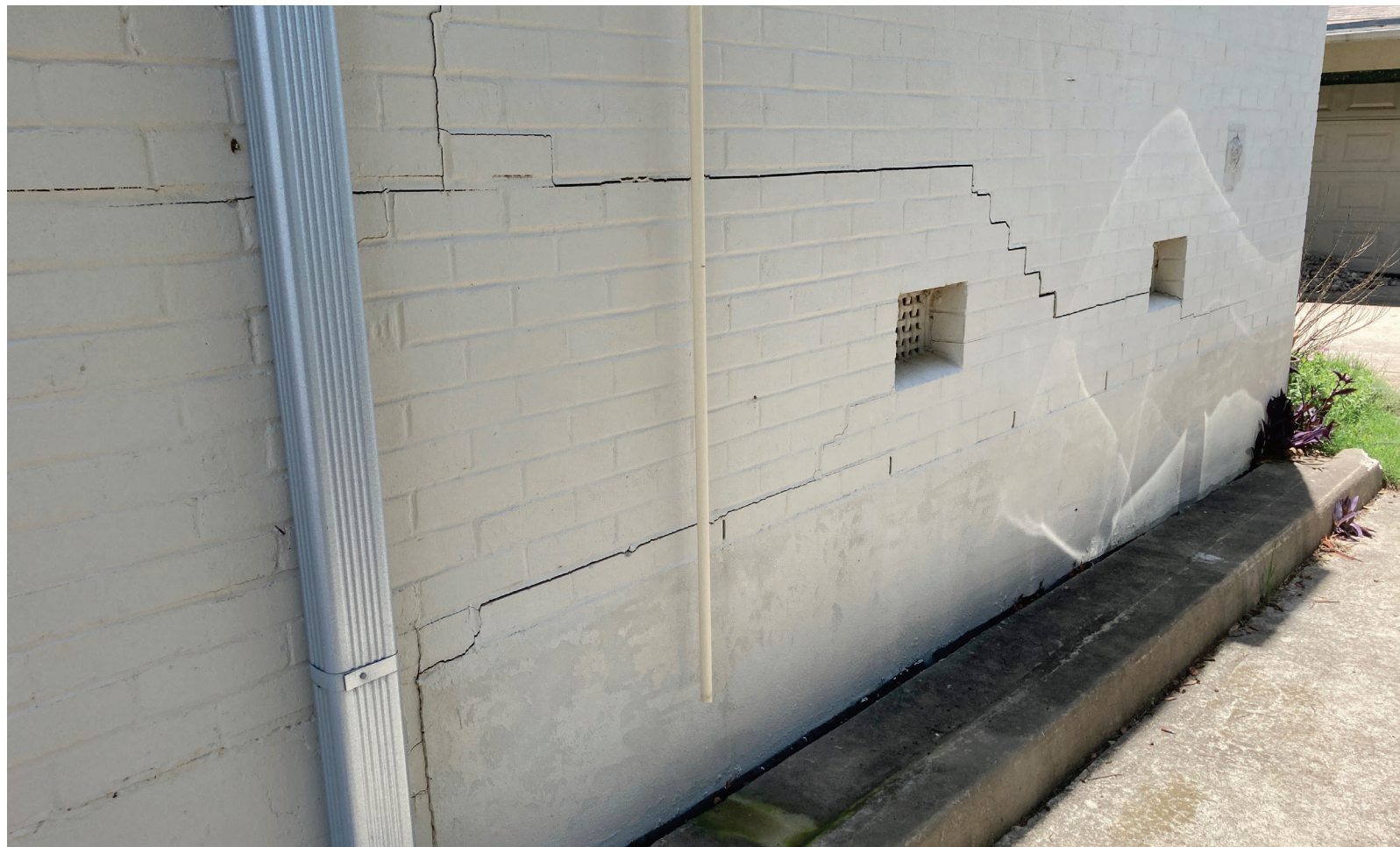
TYPICAL MASONRY CRACKS
